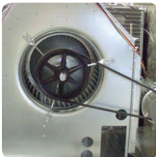
PowerMax DriveN Pulley on a Centrifugal Fan.
